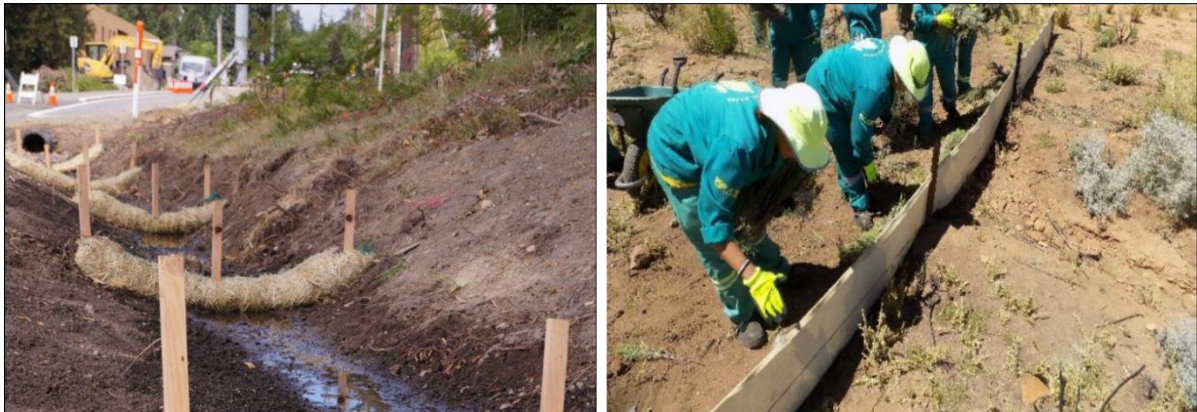
Figure 19. Examples of silt socks (left) and a silt fence (right) placed perpendicular to the flow of water. These methods reduce the force of water flow, erosion and can prevent unwanted sedimentation a site.
