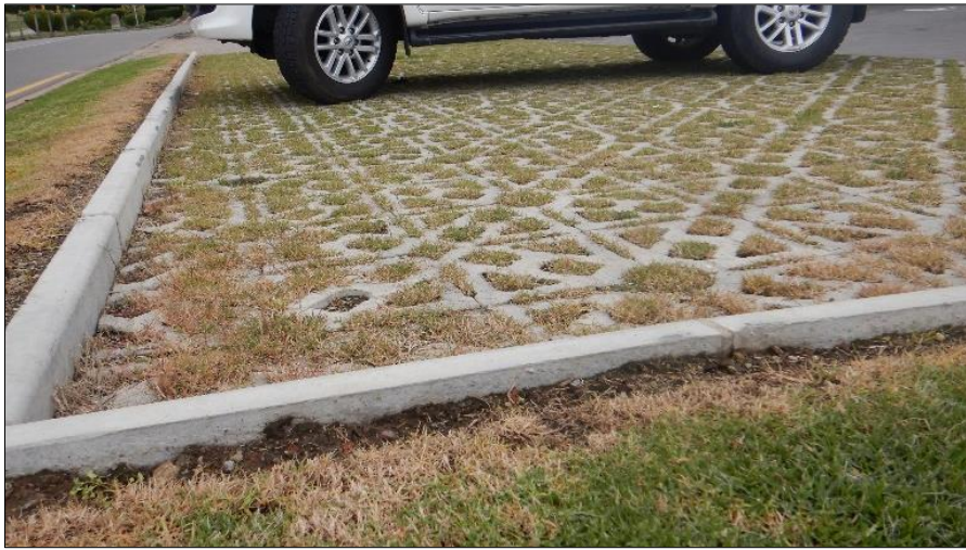
Figure 17. Examples of open pavers to improve water infiltration and prevent soil erosion.
