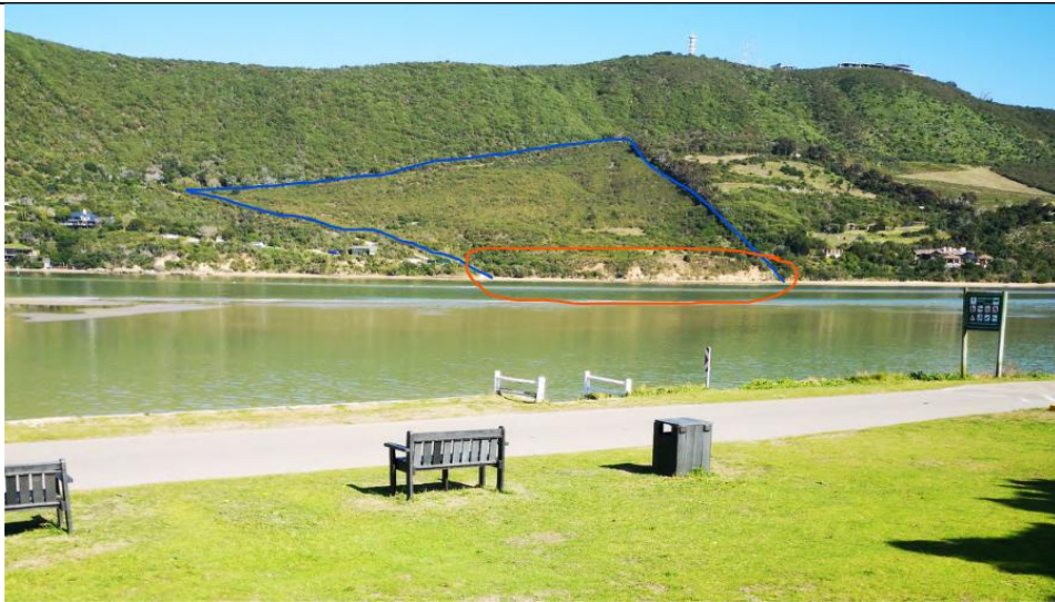
Figure 3: Image from the BAR indicating the exposed and eroded steep dune of the property.
