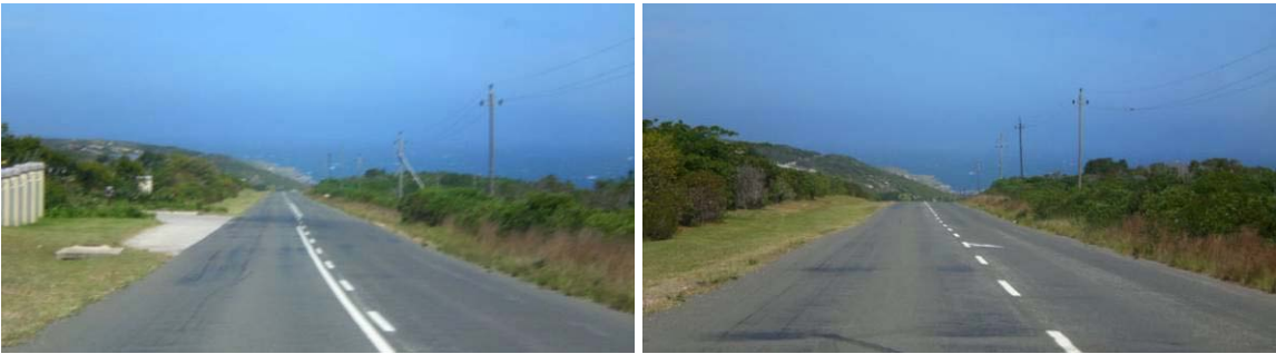
Figure 7: Looking south down Robberg Road with the property on the right
