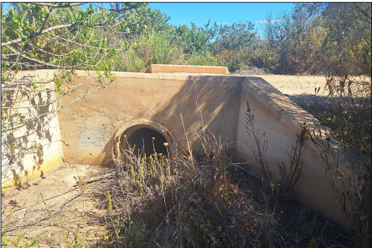
Plate 3: Photograph of the road culvert which is not in fact within riparian habitat but directs surface runoff, collected by the roadside ditch upslope, towards the downslope watercourse
