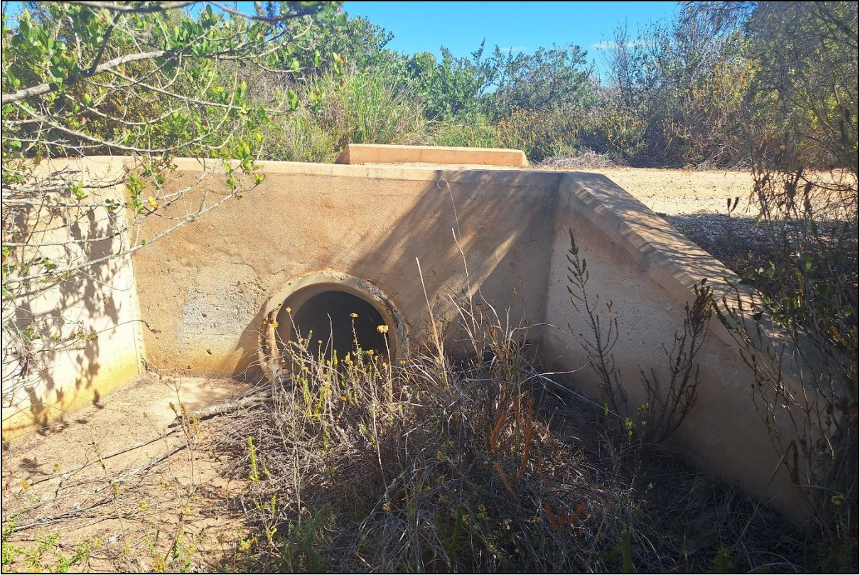
Plate 3: Photograph of the road culvert which is not in fact within riparian habitat but directs surface runoff, collected by the roadside ditch upslope, towards the downslope watercourse
