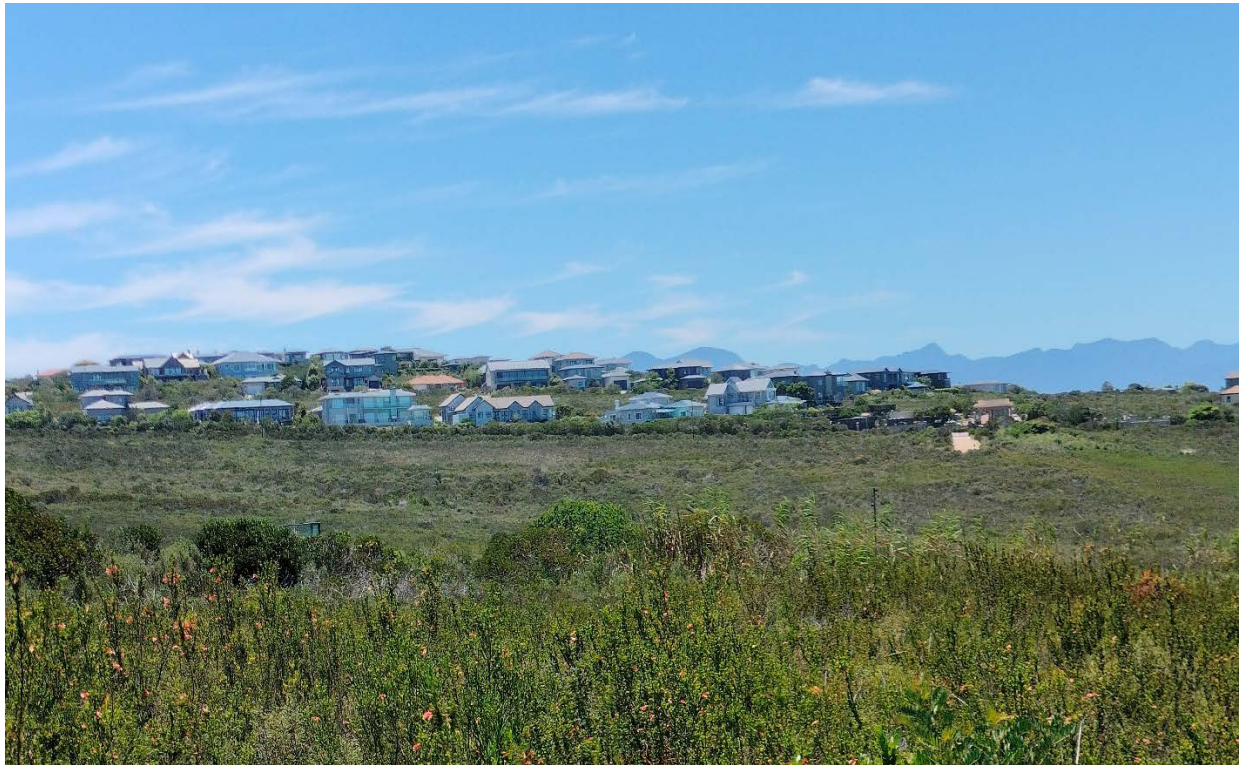
Photo 16: Taken from the quarry on Portion 63 towards Whale Rock Drive, showing the Portion 59 in the middle and Whale Rock Estate in the background
