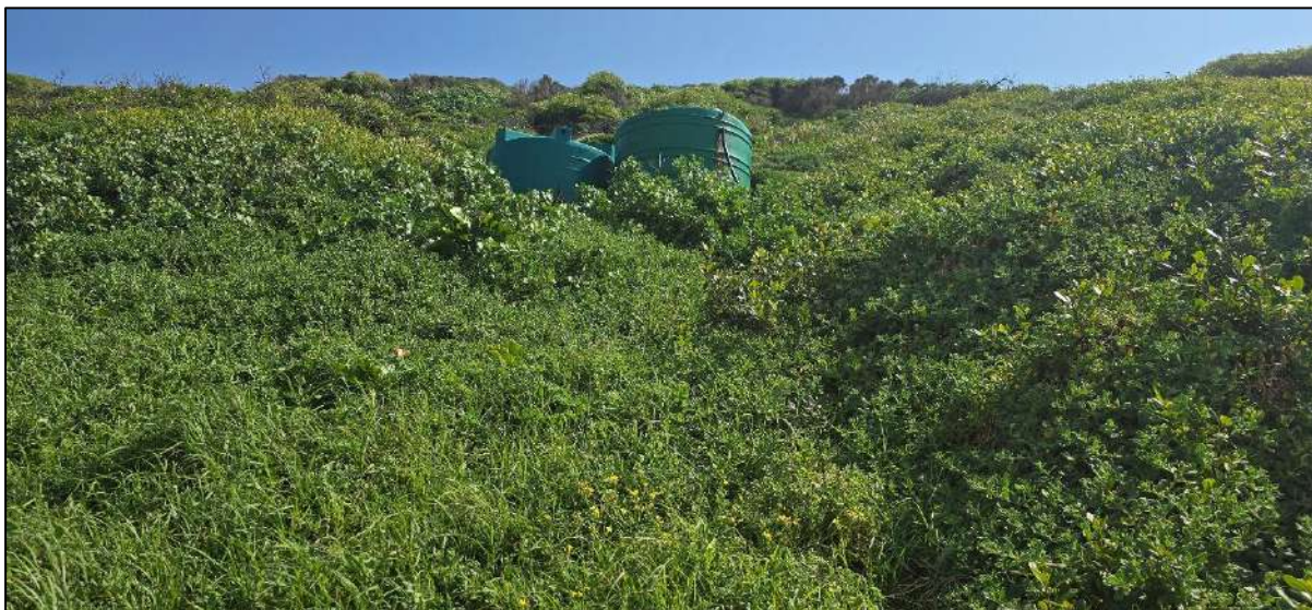
Figure 13. Associated JoJo water storage tanks that supplies the dwelling.
