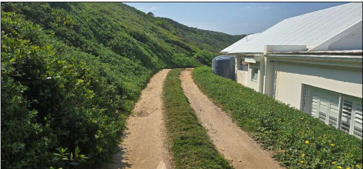
Figure 12. View of the road constructed behind the dwelling.
