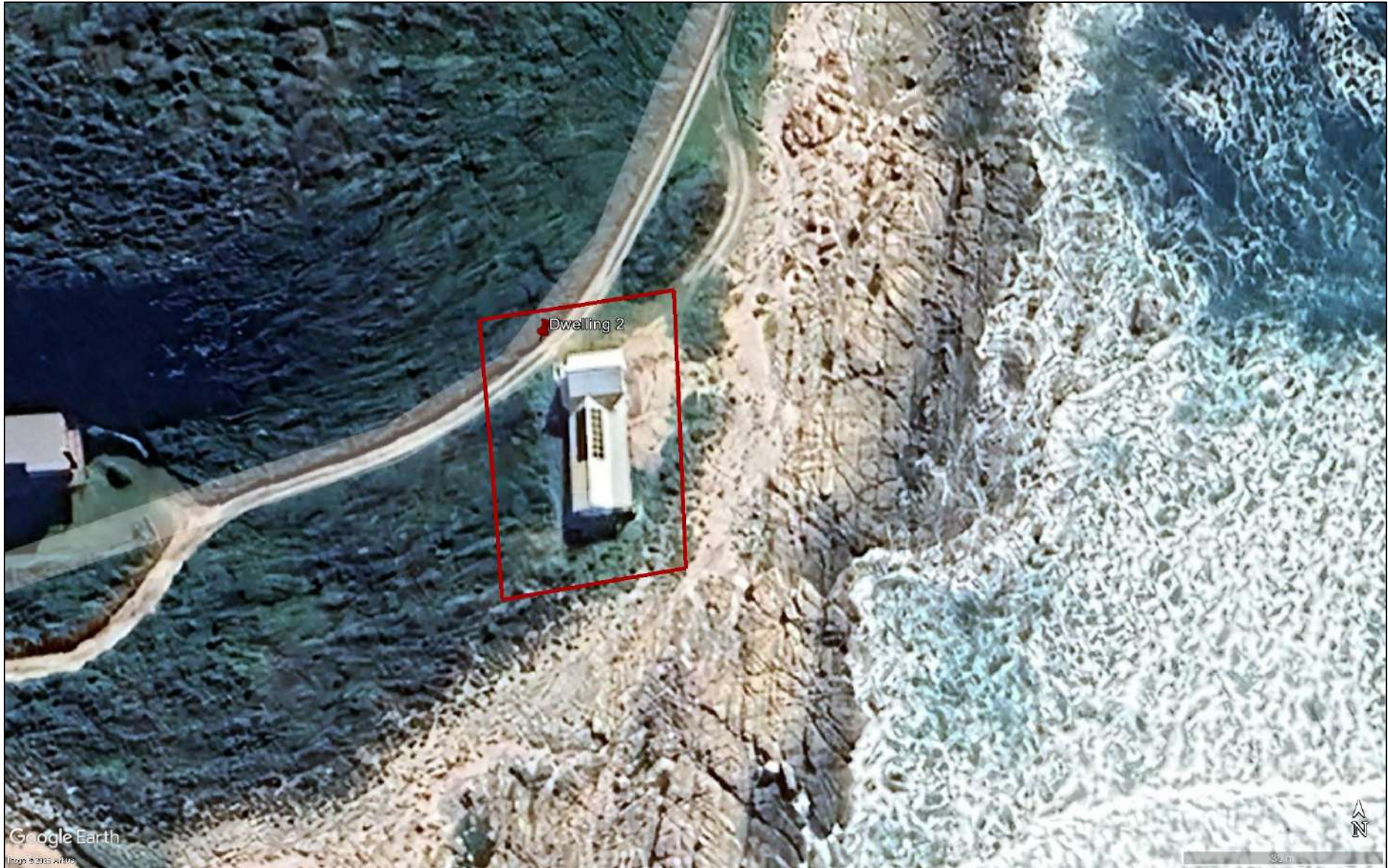
Figure 7. Close-up view of Dwelling 2 for S24G application on Portion 12 of Farm Ongegunde Vryheid No.746, Cape St Francis Bay, Kouga Local Municipality, Eastern Cape Province.
