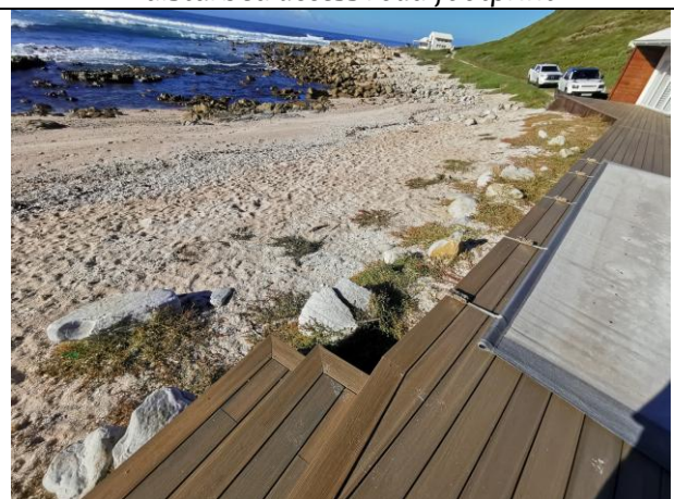
Figure 15: Front deck on edge of historically disturbed access road footprint.
