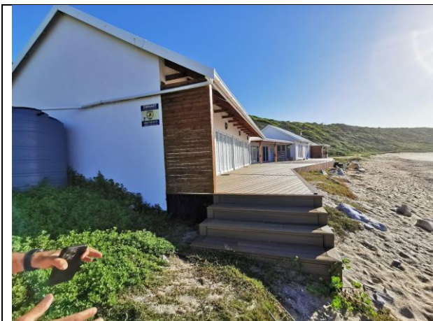
Figure 12: Front deck on edge of historically disturbed access road footprint
