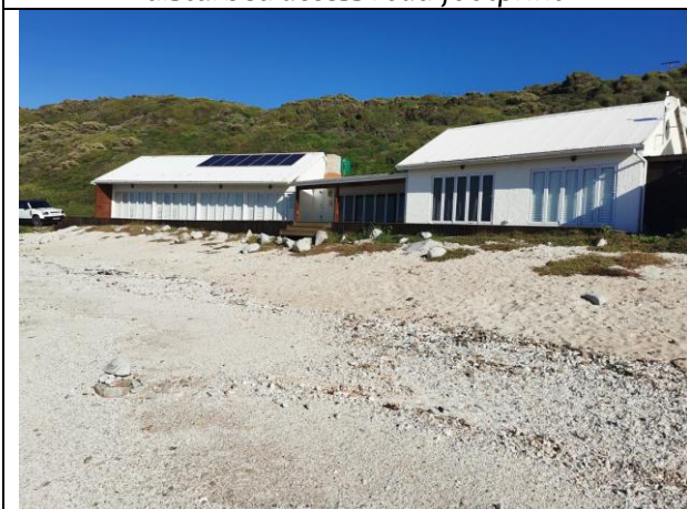
Figure 14: Front deck on edge of historically disturbed access road footprint.
