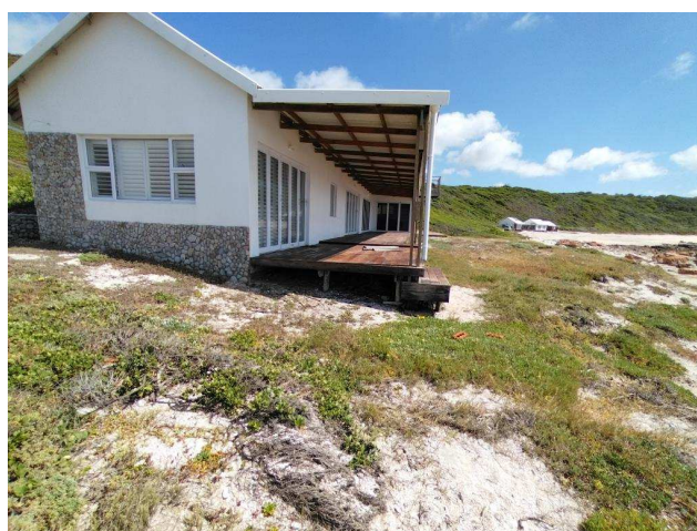
Plate 4. Dwelling 2 seen from the south.
