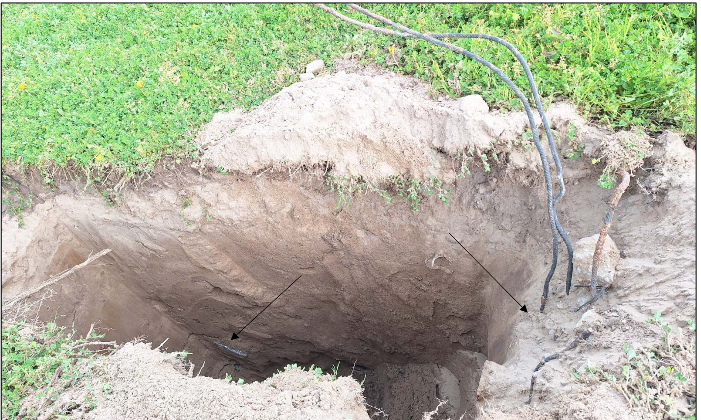
Figure 4: Rubble and remnant foundation structures encountered in some pits
