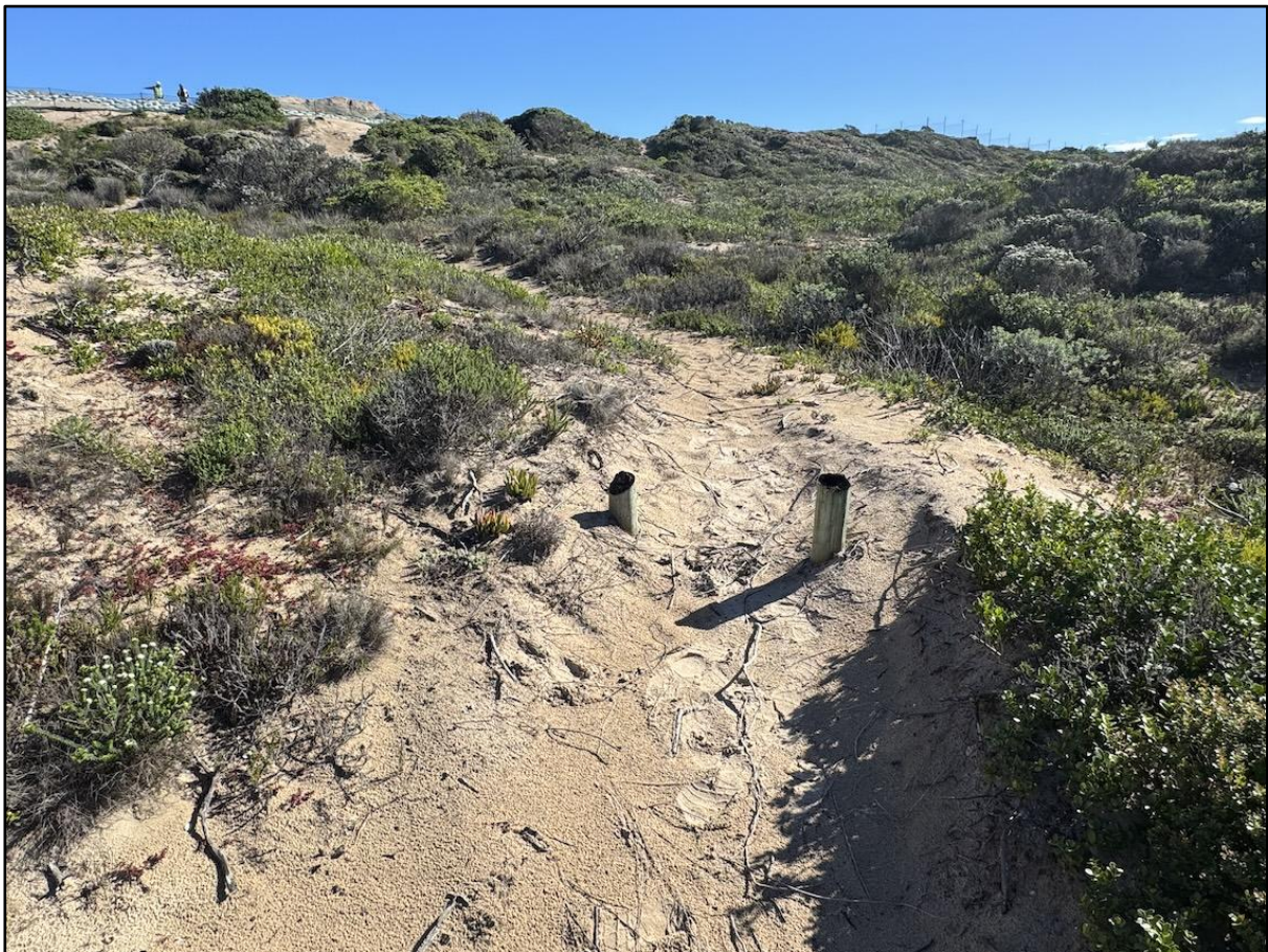
Figure 9: Previous location of boardwalk, lost during fires of 2017 (old support poles still visible).
