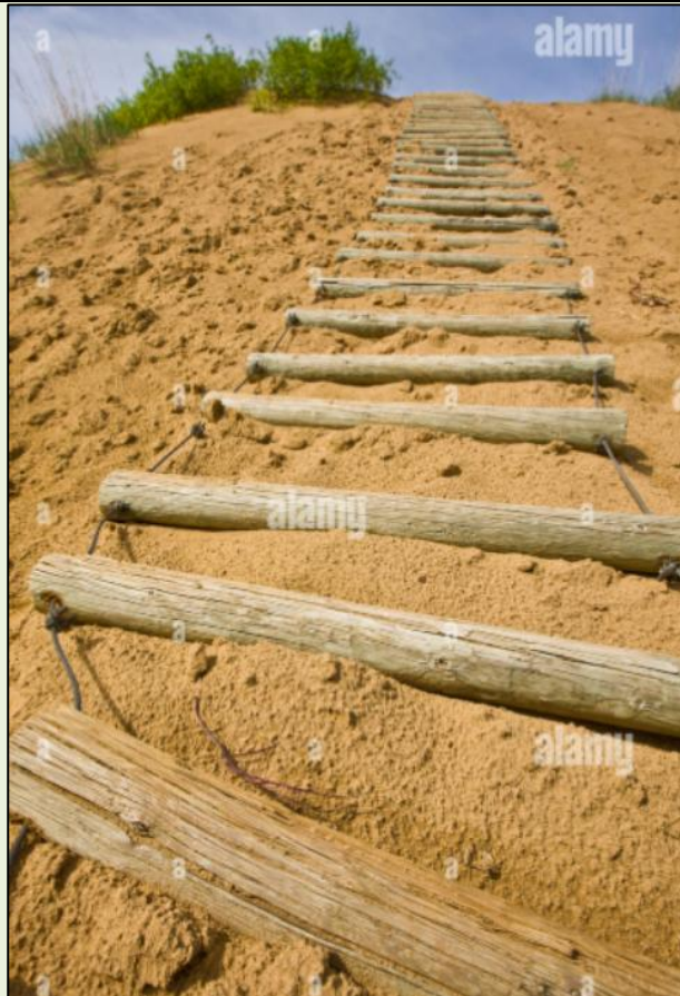
Figure 2: Example of soft engineering method
