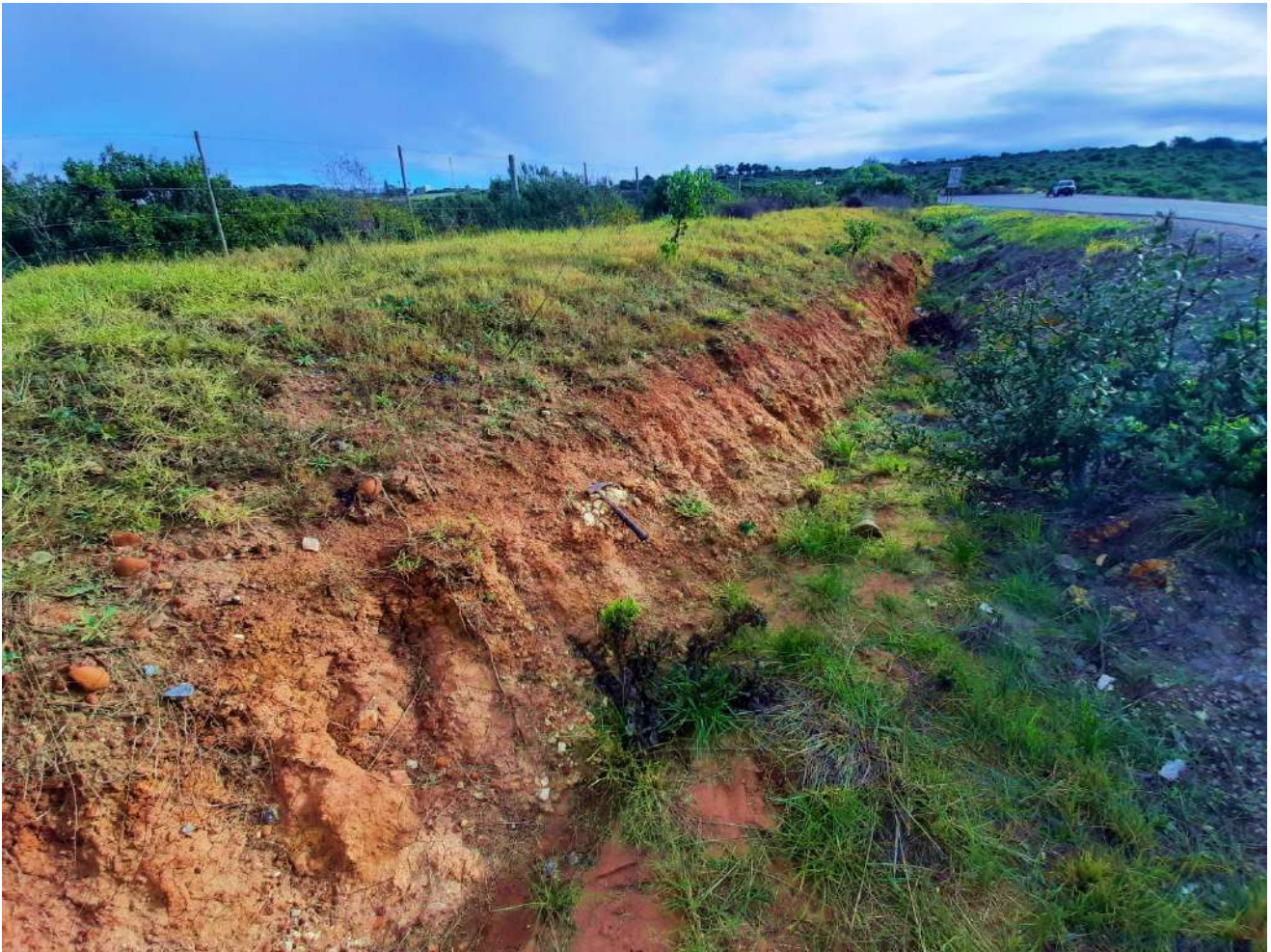
Figure 15. the drainage ditch next to the road, exposing some weathered Enon Formation.
