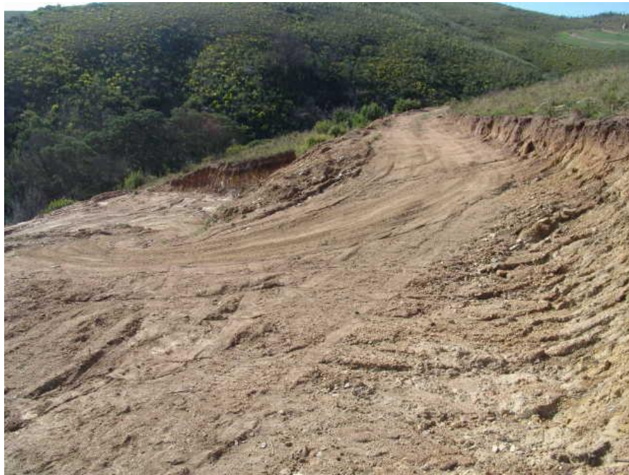
Photo 3: Bends in the steep section of the upgraded road at Site 5. Note the soil erosion from these fragile granitic soils.
