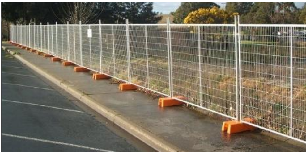
Figure 22. Example of construction fencing to be used to demarcate construction areas.
