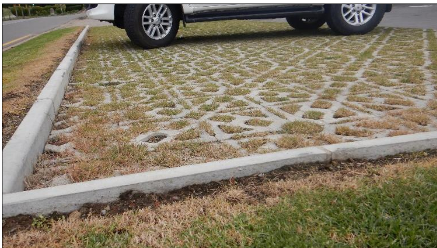
Figure 21. Examples of open pavers to use for parking areas, access roads or underneath gutters/water tank overflow areas to improve water infiltration and prevent soil erosion.
