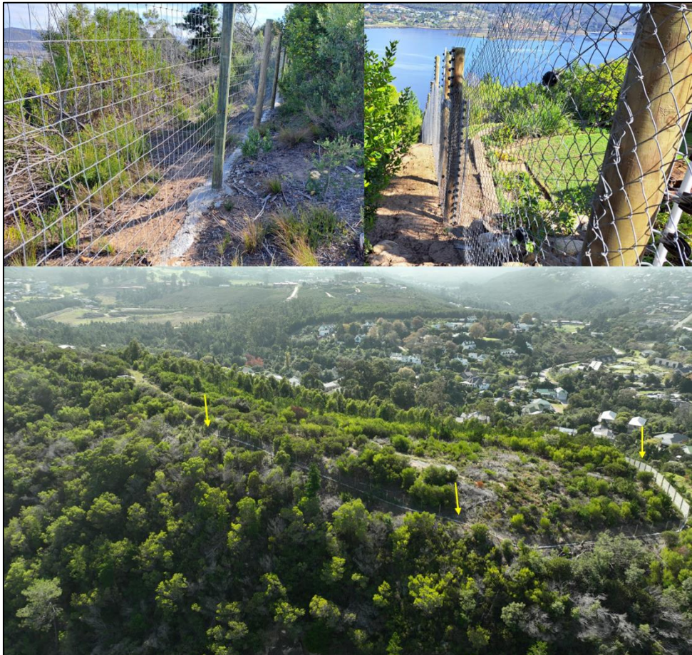
Figure 15. Fencing seen along some sections of Erf 2925, extending to Erf 2924 on the hilltop (top left and bottom image). The neighbouring property to Erven 7594 and 2924 also has a fence line with numerous and very tightly spaced electric wires (top right image).
