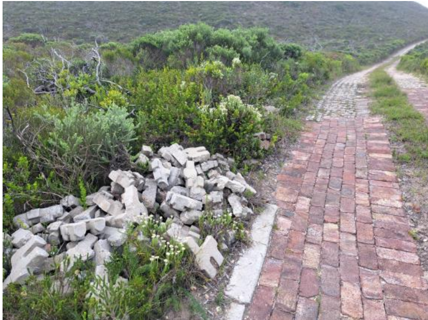
Figure 26. Inappropriate disposal or storage of pavers used during road maintenance activities.
