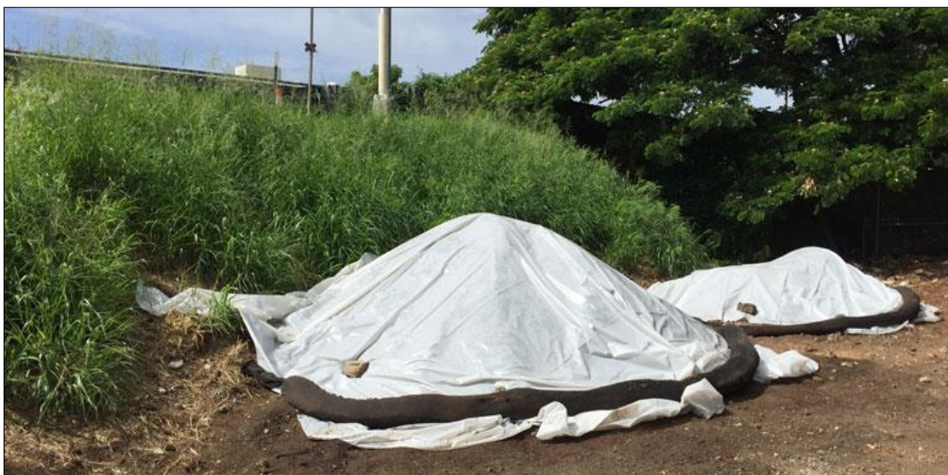
Figure 24. Stockpiles of fine textured building materials and soils covered with geotextile/plastic covering and bunded with sandbags when not in use.
