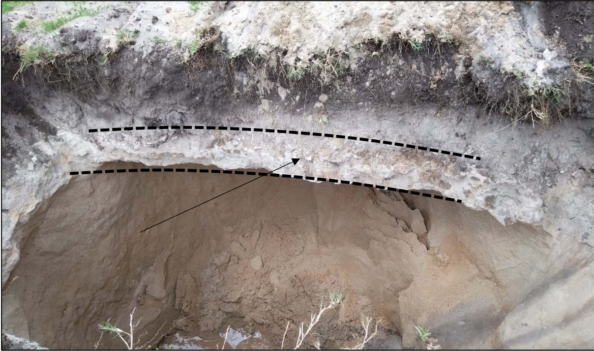
Figure 7: Calcrete hardpan layer encountered in test pit TP5
