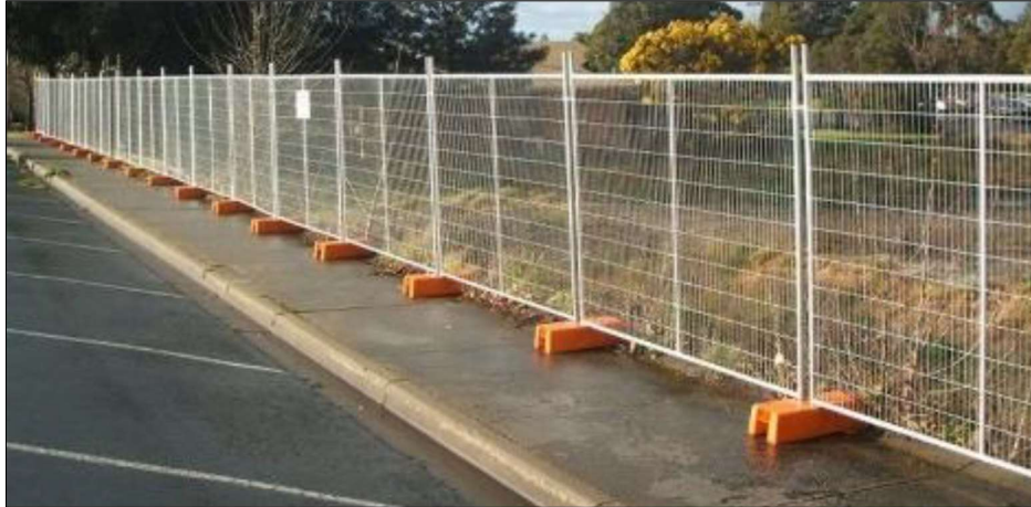
Figure 20. Example of construction fencing to be used to demarcate construction areas.
