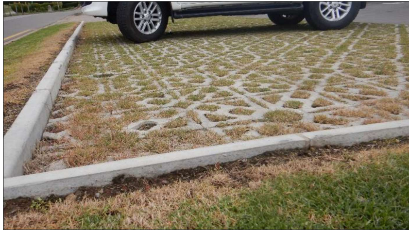
Figure 19. Examples of open pavers to use for parking areas, access roads or underneath gutters/water tank overflow areas to improve water infiltration and prevent soil erosion.
