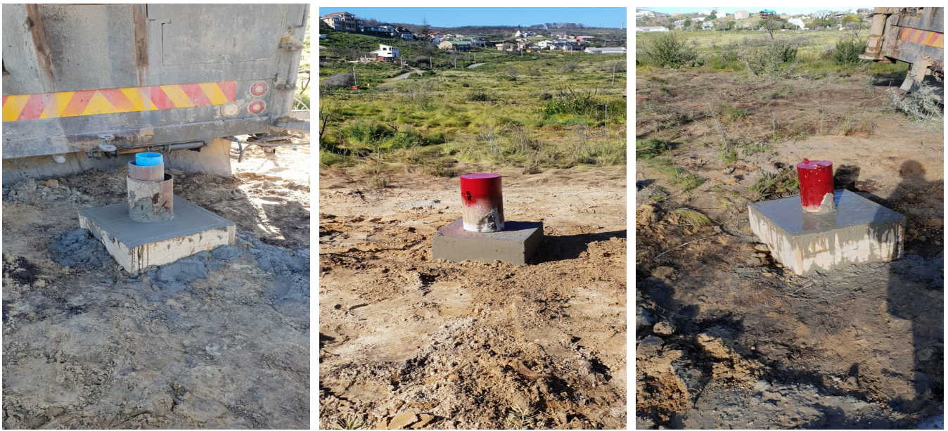
Plate 2 – Completed boreholes with lockable cap and concrete collar on Ptn 71 & 72.
