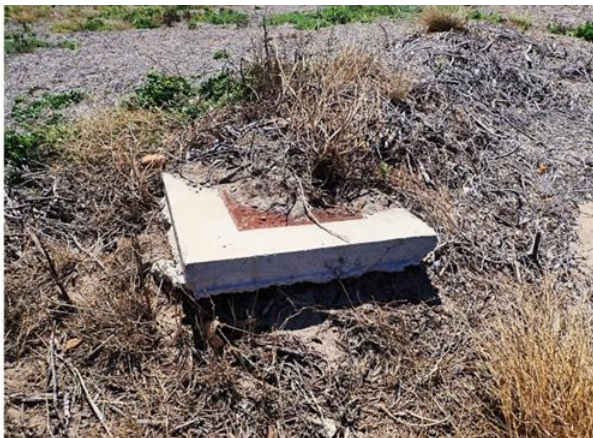
Figure 4: Bulk service installed on site prior to March 2006.
