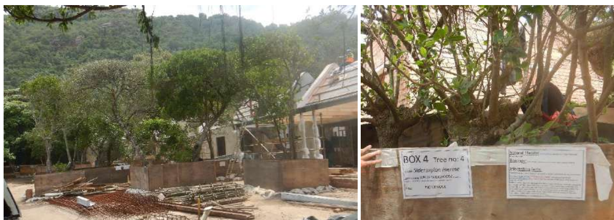
Figure 10: An example of a construction site with protected and other indigenous trees marked and sectioned off from the rest of the construction site. Each tree and box was marked, and interesting facts about the species and its ecology was provided on the construction site.
