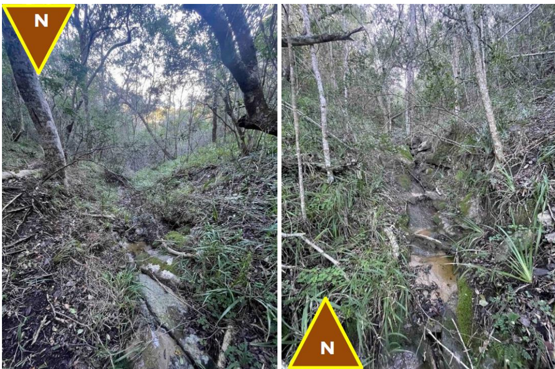
Figure 15: The eastern drainage line of Erf 301. The direction faced is indicated on the images with a North arrow. Photos taken by the owner.
