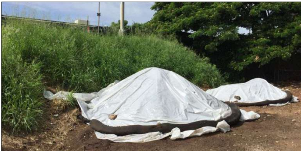
Figure 22. Stockpiles of fine textured building materials and soils covered with geotextile/plastic covering and bunded with sandbags when not in use.
