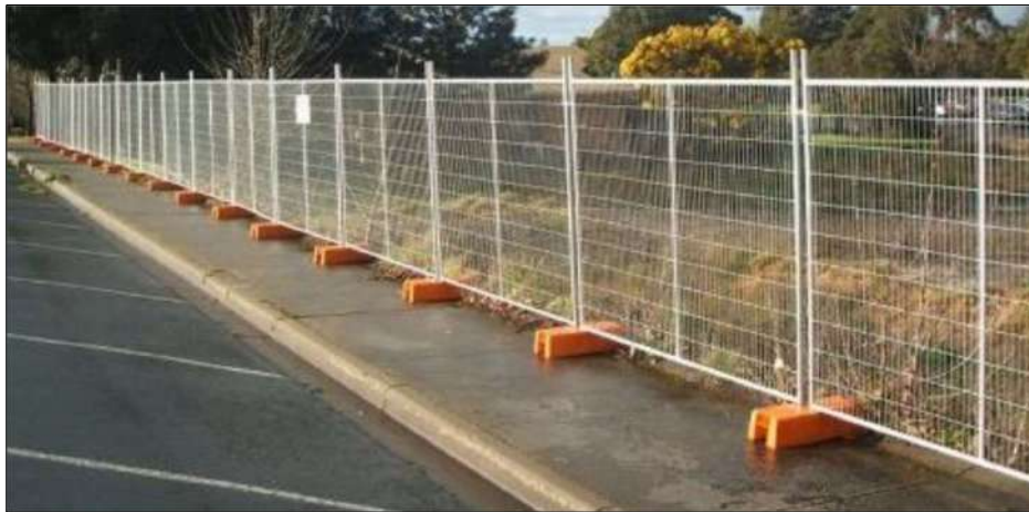
Figure 21. Example of construction fencing to be used to demarcate construction areas.
