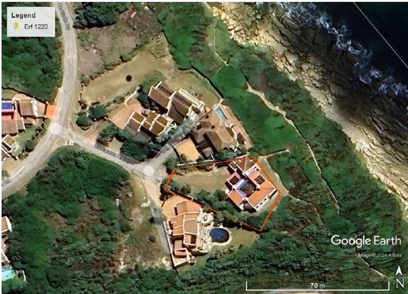
Figure 2: Erf 1120 located with 100 meters of the high-water mark of the sea
