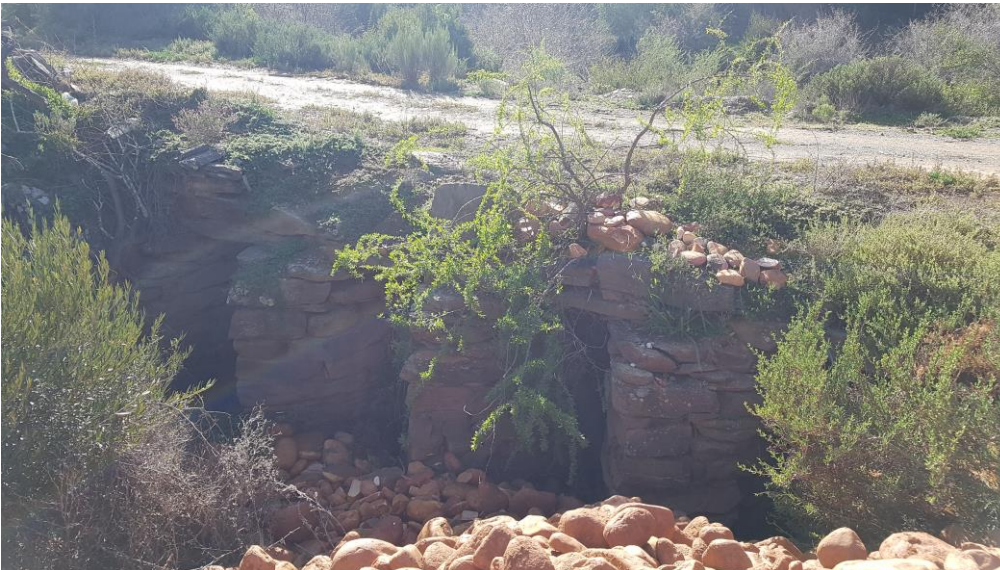
Figure 7: Existing access to dam wall over historical river crossing.
