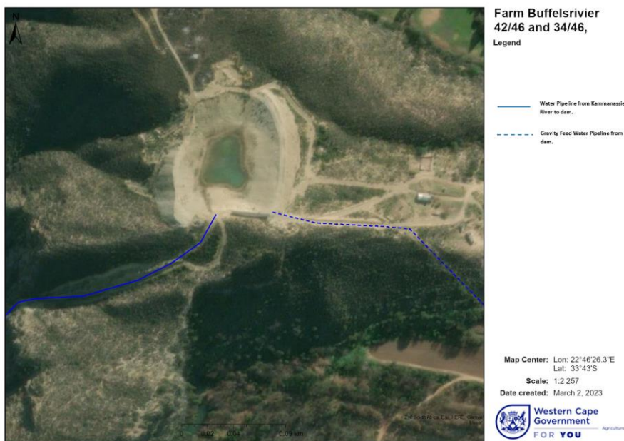
Figure 9: Water Pipelines for Kop Dam.
