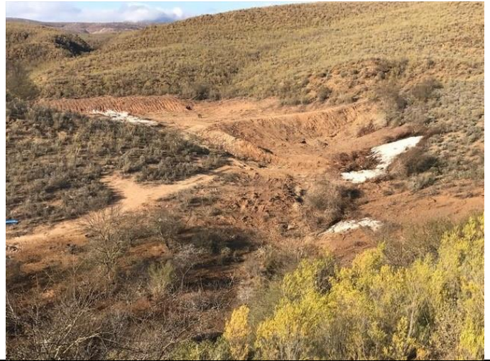
2. Area where dam wall was constructed.
