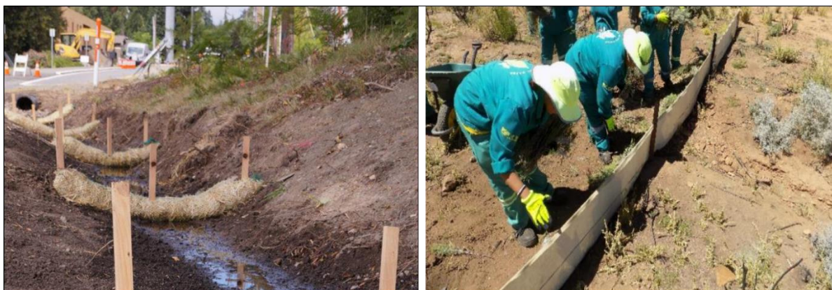
Figure 17. Examples of silt socks (left) and a silt fence (right) placed perpendicular to the flow of water. These methods reduce the force of water flow, erosion and can prevent unwanted sedimentation a site.
