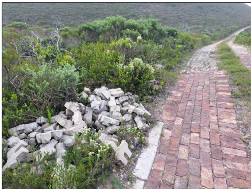
Figure 20. Inappropriate disposal or storage of pavers used during road maintenance activities.
