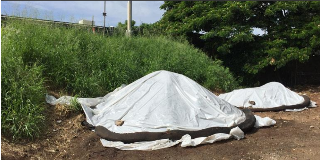
Figure 18. Stockpiles of fine textured building materials and soils covered with geotextile/plastic covering and banded with sandbags when not in use.
