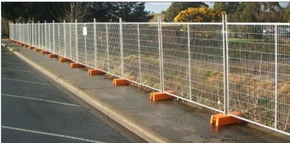
Figure 16. Example of construction fencing to be used to demarcate construction areas.
