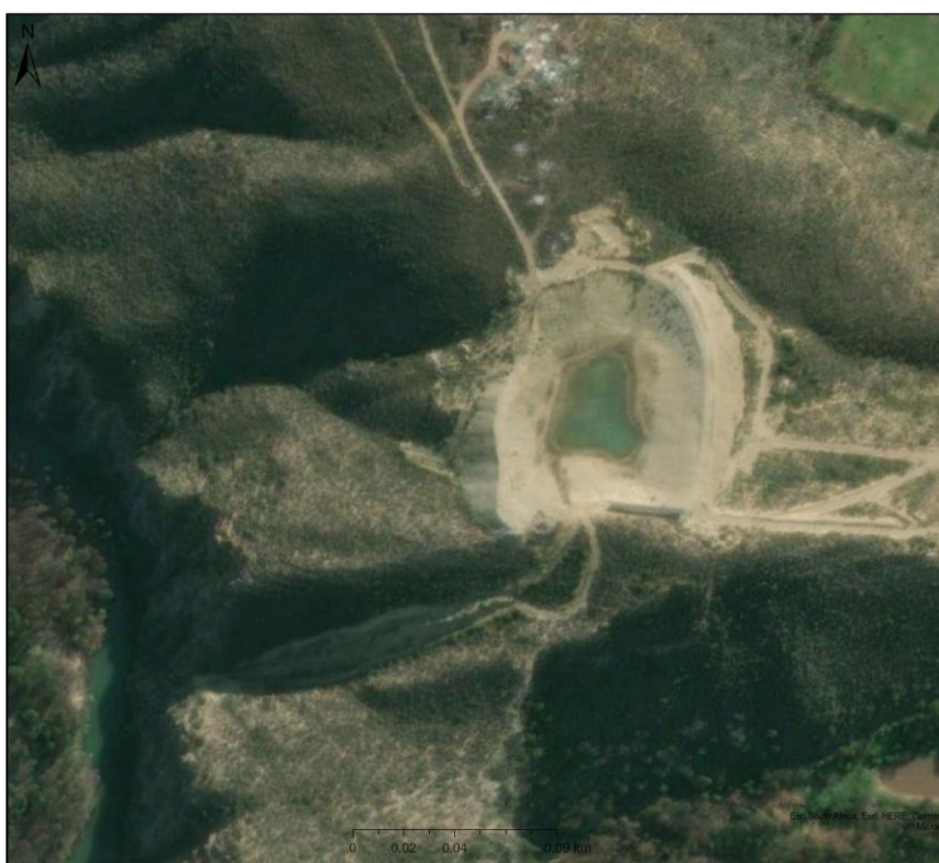
Figure 2: Location of Kop Dam post-construction.
