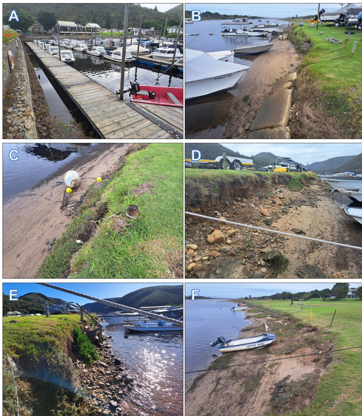
Figure 11: Photographs illustrating existing gabions and jetties at the PBAC (A); boats mooring along the eroded bank (B); actively eroding banks (C to E); and the estuary banks further downstream where erosion is not as severe (F).
