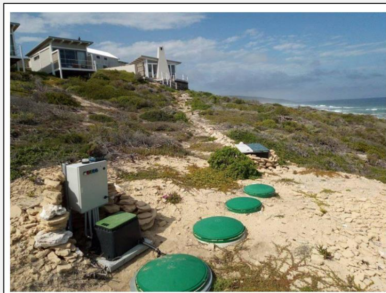
Figure 3: Clarus Fusion® installation at De Hoop Nature Reserve
