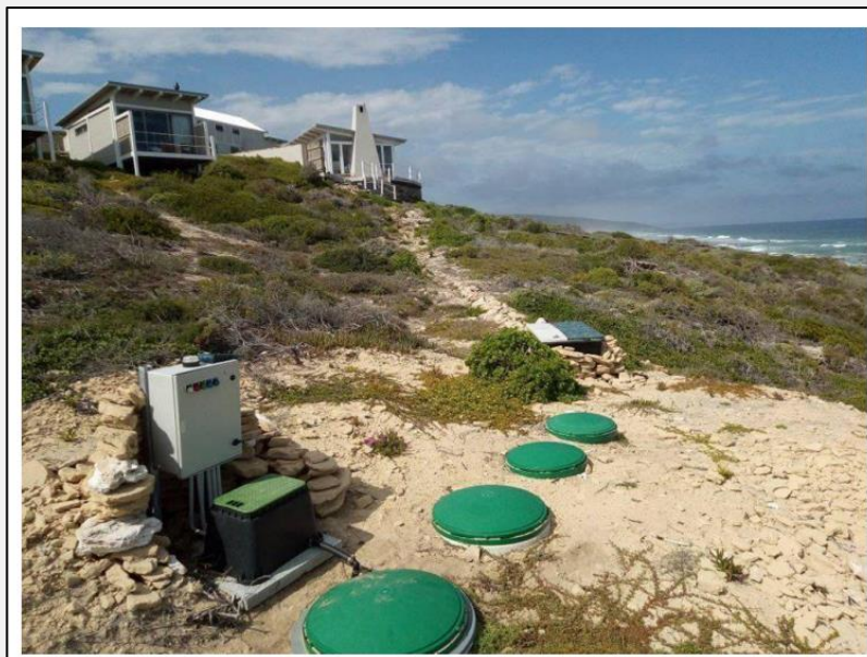
Clarus Fusion® installation at De Hoop Nature Reserve
