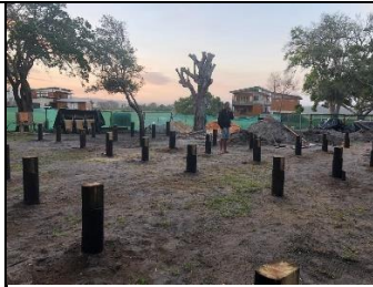
Figure 13 Pad foundations
