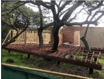
Figure 14 Tree roots were protected by pad foundations.
