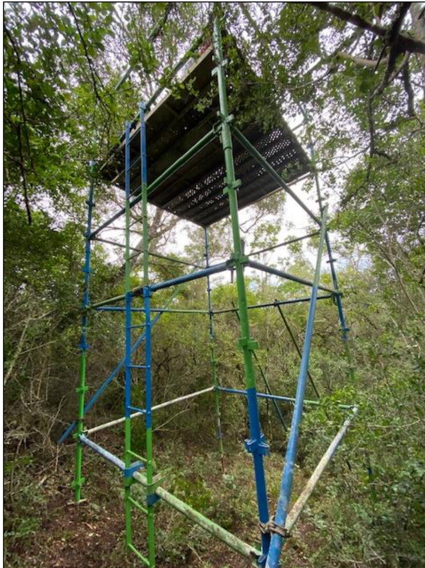
FIGURE 3: SCAFFOLDING PLACED ON SITE
