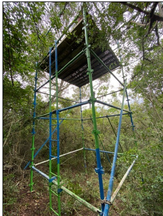
FIGURE 3: SCAFFOLDING PLACED ON SITE
