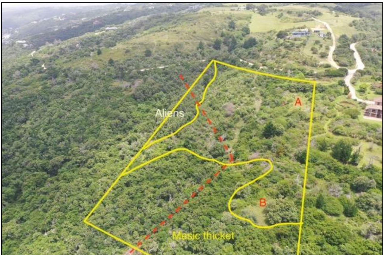
Figure 15: Drone image of the site with approximate position of boundaries shown, as well as some important features on site. The red dashed line is the powerline that crosses the site.
