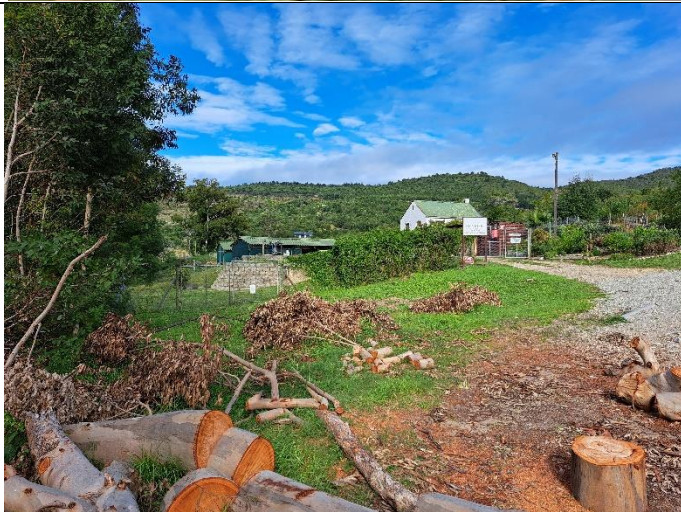
1. View of the Knysna Wastewater Treatment Works on the western boundary.
