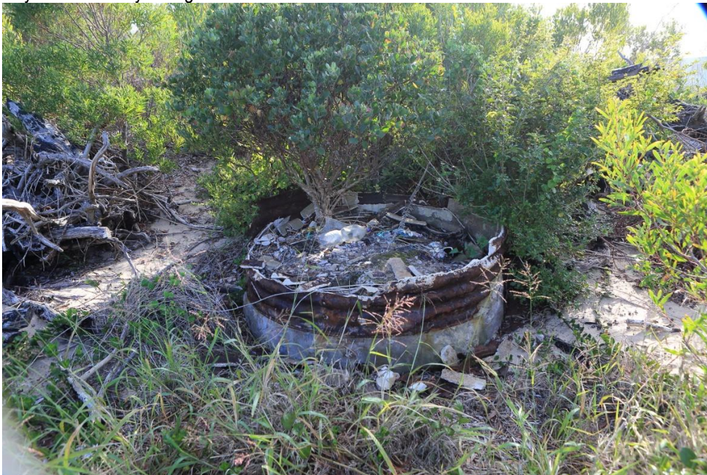
Fig-7: Water tank
