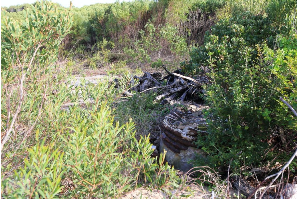
Fig-8: Concrete Slab
