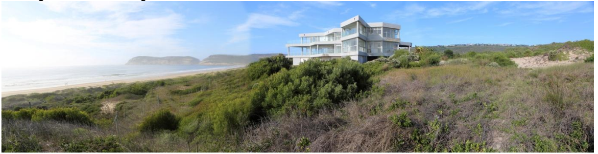
Fig-10: Views towards the East and the South.
