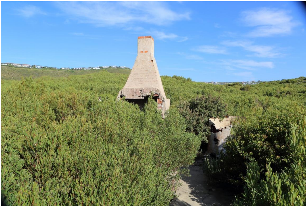
Fig-9: Fireplace, flue, water tanks and concrete slab
