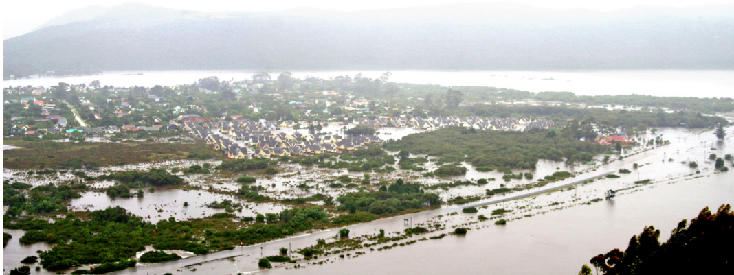
Photograph C4. November 2007: Low lying areas flooded, high lying areas not flooded
