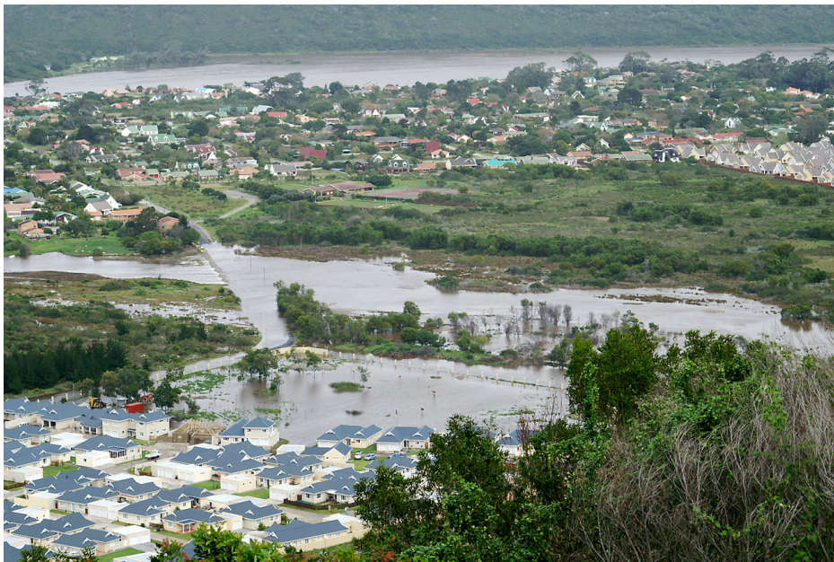
Photograph C2. August 2006: the Perdespruit causeway backs up water upstream to Montage Village and erf RE1627
