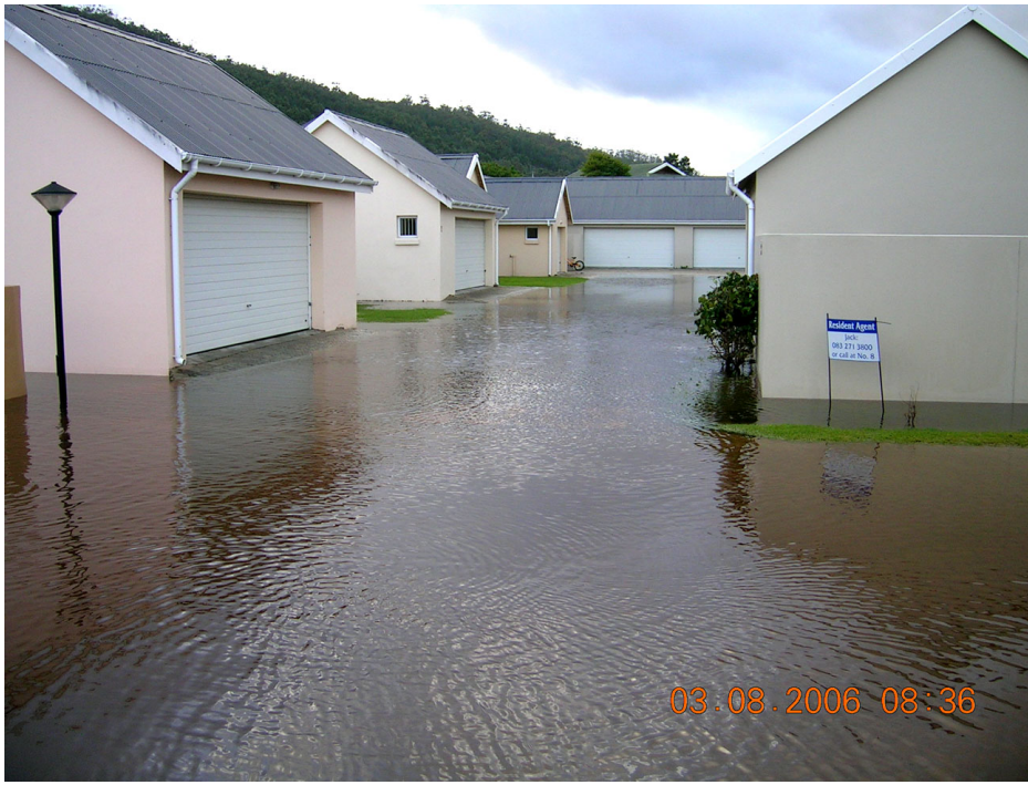
Photograph C1. August 2006: Montage Village flood levels below the 3.0m amsl floor levels.
