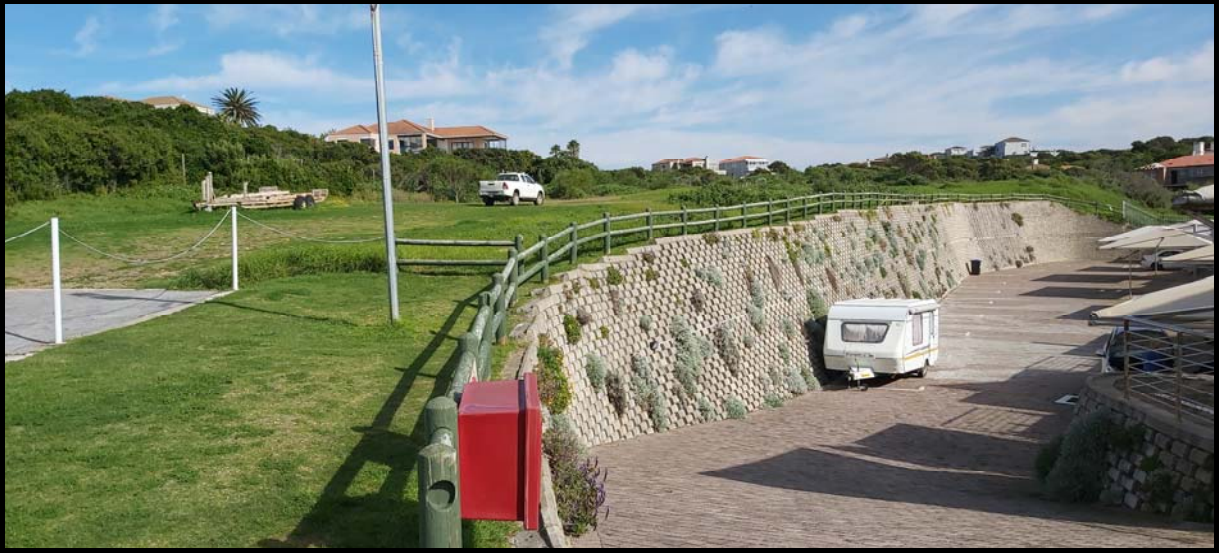
Figure 4: View of the retaining wall along the northern boundary, looking to the west
