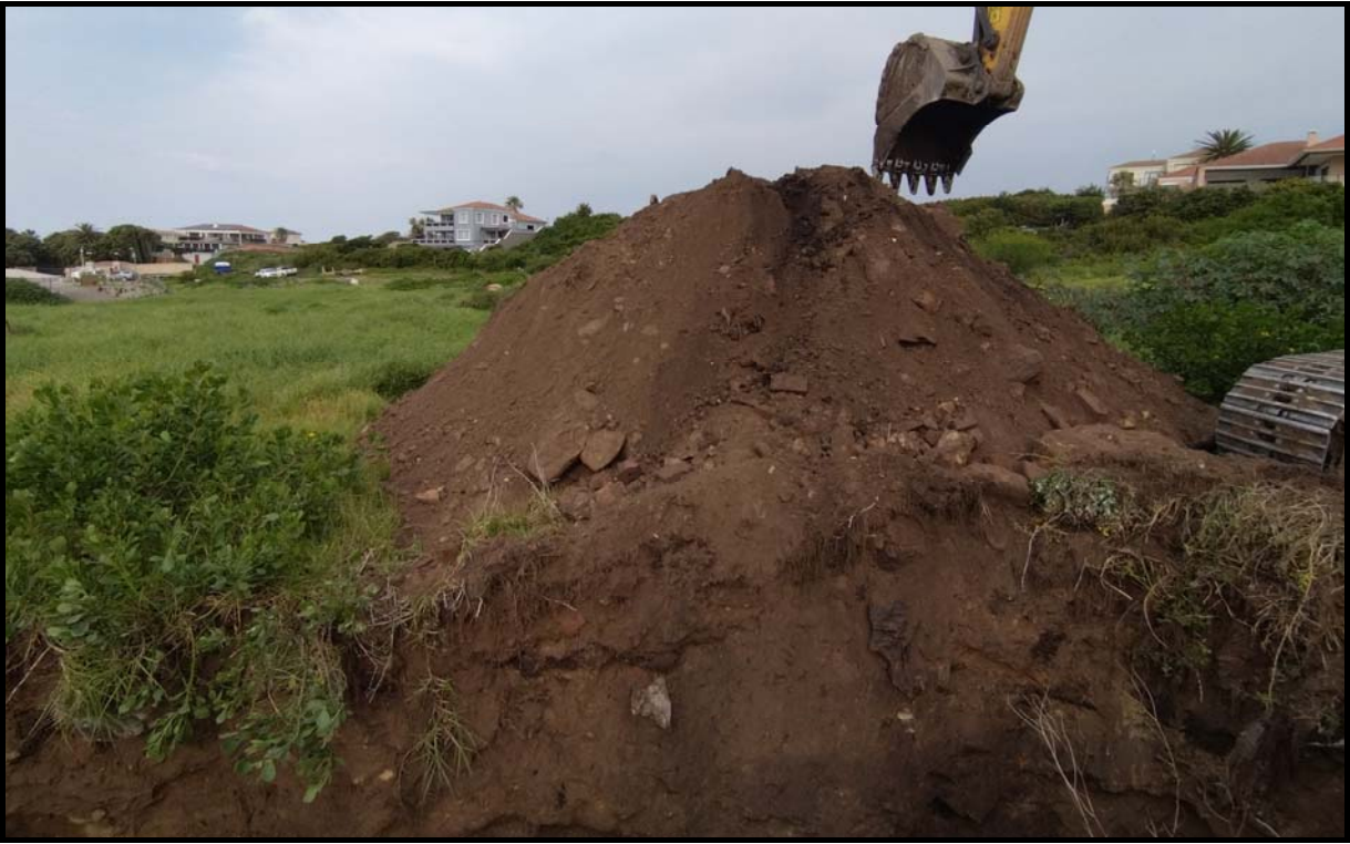
Figure 9: Gravelly sandy fill material encountered below surface in all pits
