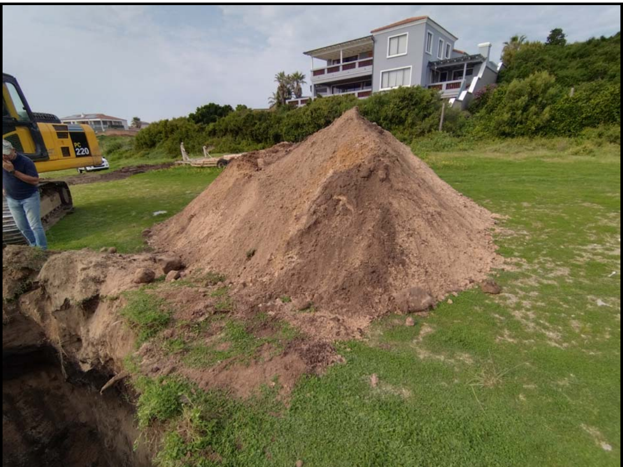
Figure 10: Typical insitu aeolian silty sand encountered in the test pits
