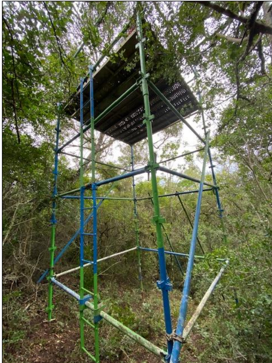
FIGURE 3: SCAFFOLDING PLACED ON SITE
