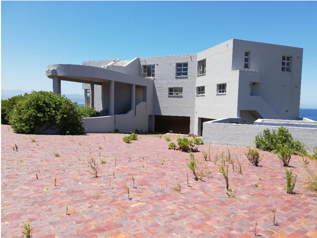
Figure 3: Existing Structure on Portion 66
