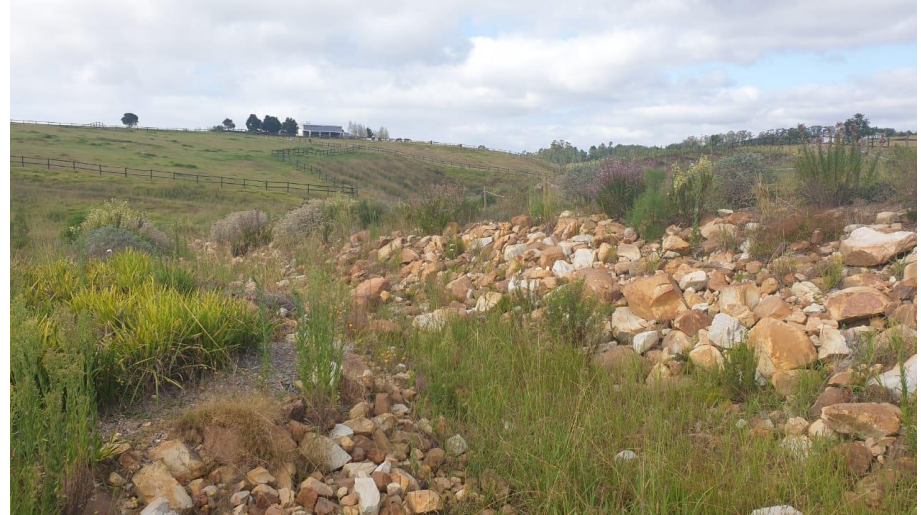
Erosion rehabilitation and prevention
