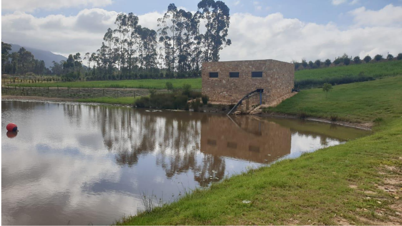
Dam 2 (Portion 66) and pump house.
