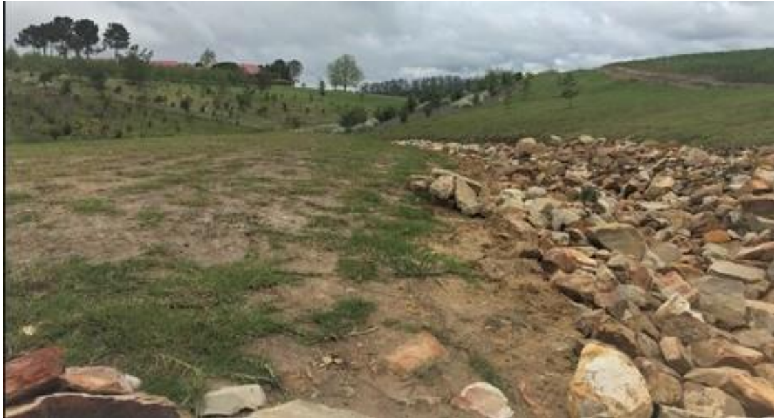
Figure 12: Showing the rock infilled watercourse (erosion prevention by landowner) at the low water crossing draining towards Dam 1.
