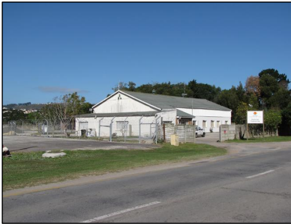
FIGURE 23: KNYSNA MUNICIPALITY ELECTRICAL DEPARTMENT.
