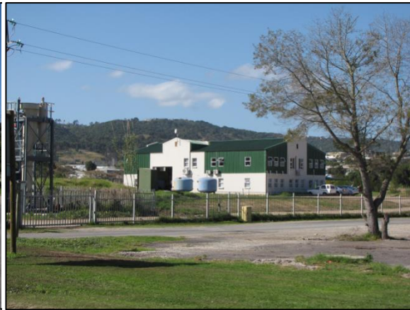
FIGURE 24: MUNICIPAL REVERSE OSMOSIS FACILITY.
